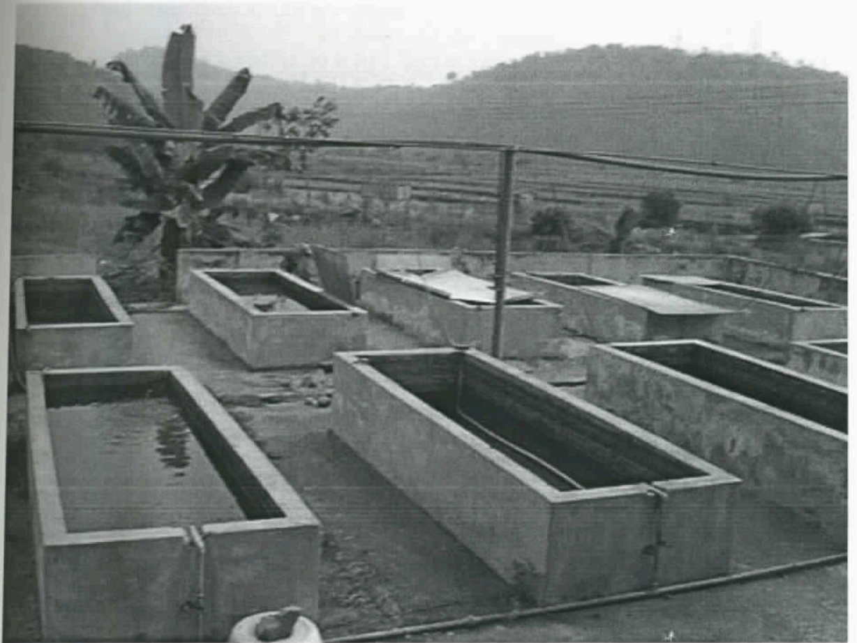
Plate 2 : Outdoor concrete tanks for rearing fry.
