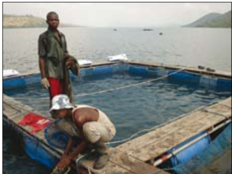
Decking attached with U-bolts to the metal pipe frame facilitates working around the cage.
