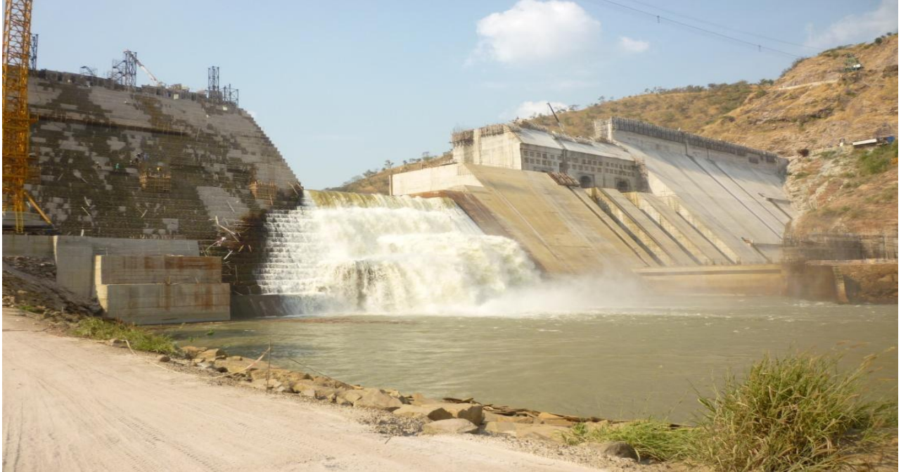
Plate Q: A view of the early spill-over at the Bui dam (Picture taken, November 2011)
