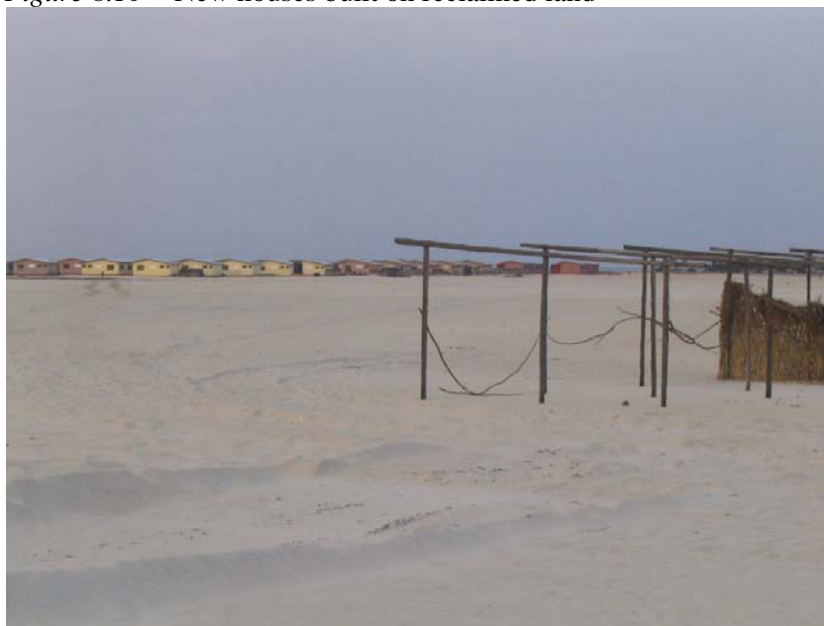
Figure 8.10 New houses built on reclaimed land
